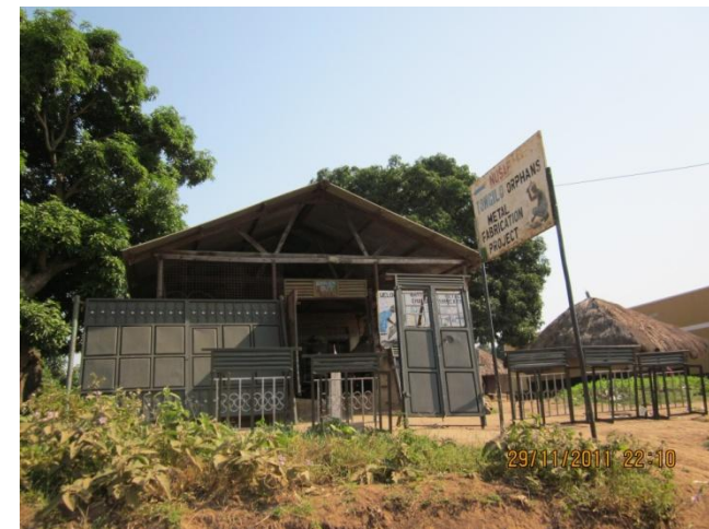
Picture 47: Training facility in Arua
