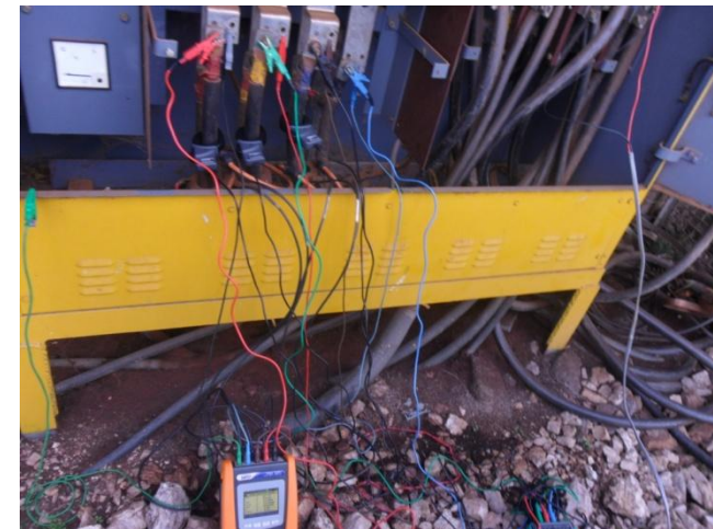
Picture 4: Energy efficiency verification measurements
