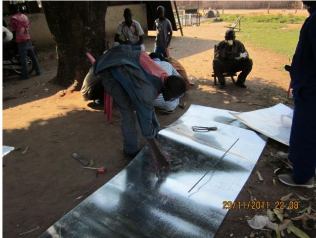
Picture 48: Measuring and cutting the metal sheet
